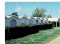
On specially shaped roof
